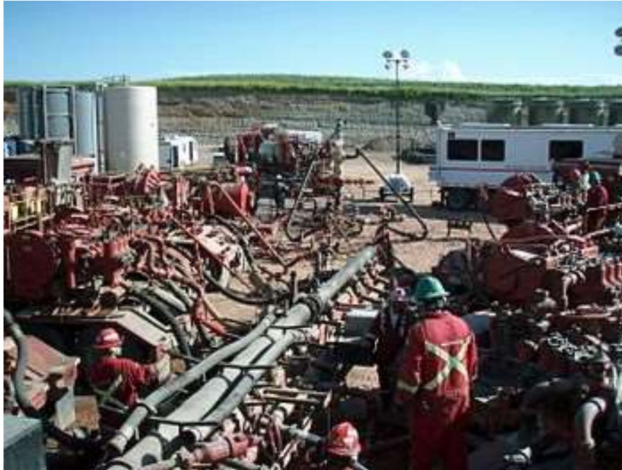
Hydraulic fracturing operations in progress
