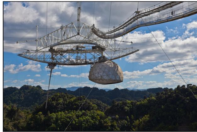
*"3918 Arecibo Observatory Beam Steering Mechanism" by Kevin Baird is licensed under CC BY-NC-ND 2.0.*
