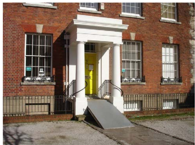
A ramp outside an old school building
